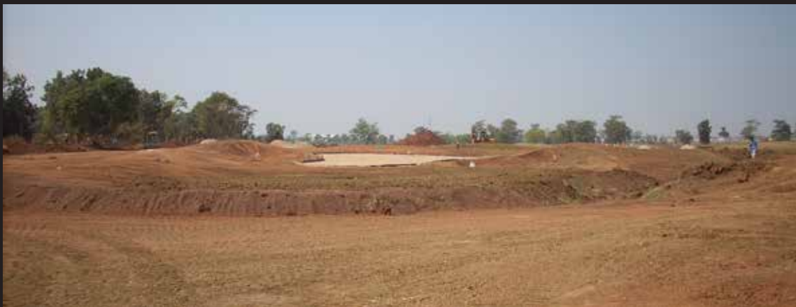
Photo Below: Construction activity at Raipur Project
